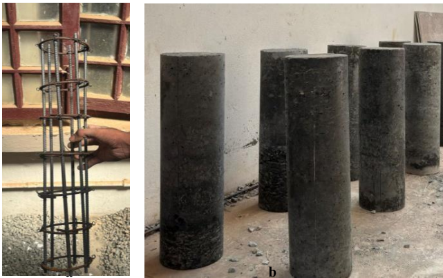
Fig. 3. (a) Reinforcement Cage and (b) Casted Columns
