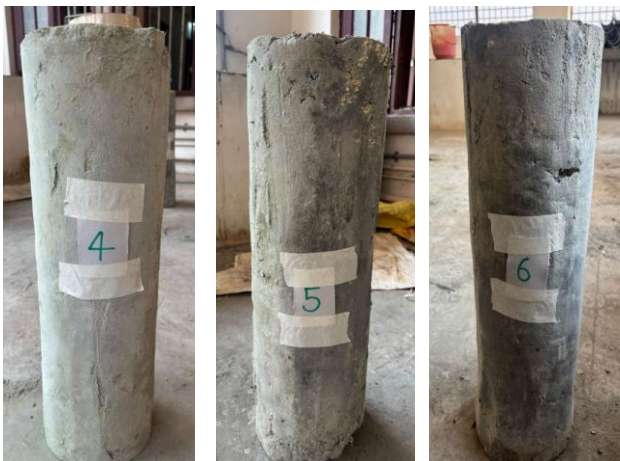
Fig. 7. Group A- Columns retrofitted with 0.5% PVA Fibre mortar mix
